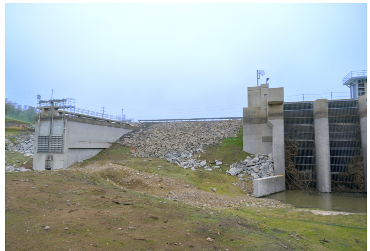
Dawson Dam automated gates.
