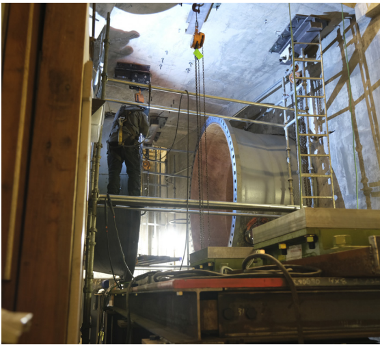
Replacement of the Turbine Shutoff Valve in Don Pedro Powerhouse.
