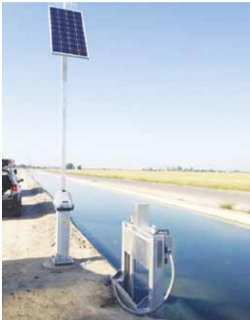
*Slip Meters like this one (accompanied by a solar-powered pedestal) will replace some sidegates within the TID system.*
