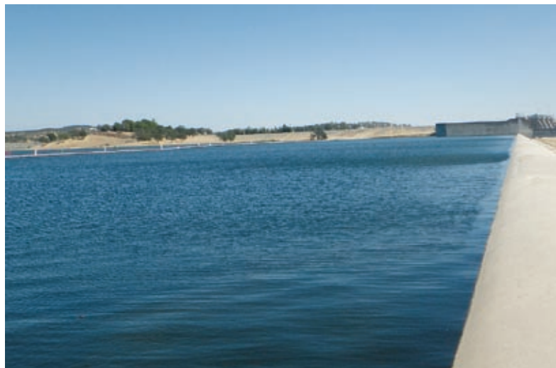
Looking south at a full Don Pedro Reservoir near the spillway.
